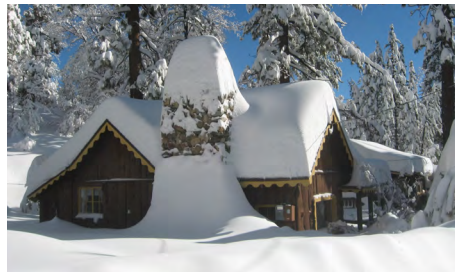
Heavy snow and ice damming can weigh down your roof potentially causing water leaks or worse.
