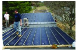
cooled system to an actively cooled system. Solar energy in the form of heat that is detrimental to the building's performance and PV performance is harvested by the thermal system and transferred off the roof portion of the building envelope into the building's domestic hot-water and radiantfloor heating system.
