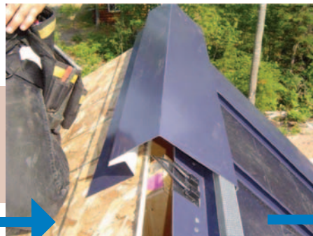
Metal roofing contractors, such as Dan Perkins of Dan Perkins Construction Inc., Ishpeming, Mich., have created and modified ridge caps to accommodate the wiring requirements of BIPV systems.
