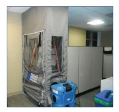
Before the physical cleaning begins, we have studied the mechanical prints and conducted a visual inspection. These are critical to understanding how the system is designed so that a plan can be outlined, access points determined, and containment protocols established.
