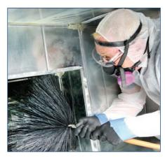
Once the section is under negative pressure, the cleaning can commence. We utilize a variety of tools depending the physical size and type of duct being serviced. Most often it's a combination of compressed air with a reverse flow nozzle and a Rotobrush application. Each section is worked towards the negative air machine, pushing dust and debris into the immense HEPA vacuum.
