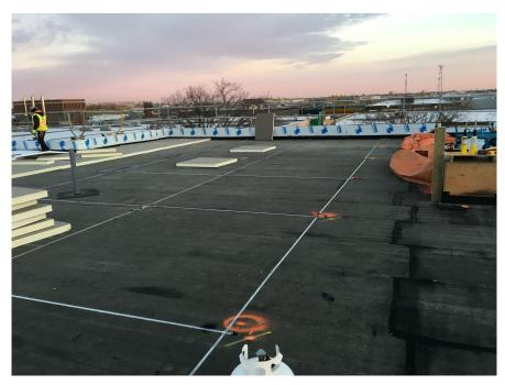
Above: FutureCast sensor grid comprises MDS tape laid out in a grid
