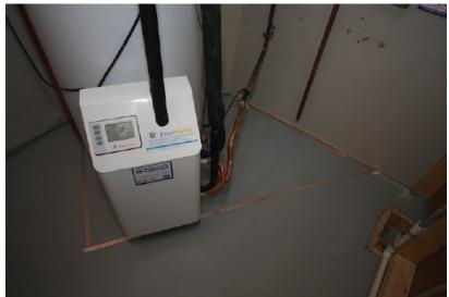
On-site monitoring is achieved through our unique wireless digital systems. These systems can be installed both during and after construction. The data gathered through these sensors will be communicated wirelessly to the Building Intelligence Gateway, which will then notify the user if necessary. This allows for facility management teams, owners, and emergency response restoration contractors to be proactive and address the situation at the very beginning.
